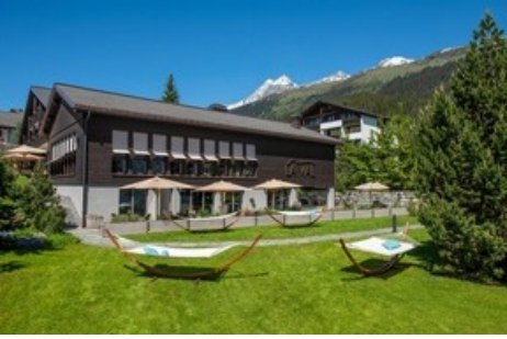
Hotel La Val, Mountain Spa, Brigels, Surselva, Switzerland. and Spa Garden
