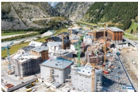
Baustelle Andermatt Reuss September 2023 © Kim Leuenberger
