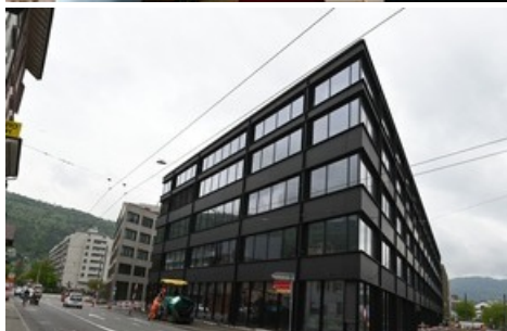
Switzerland Innovation Park Biel/Bienne SIPBB
